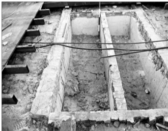
Excavations: The vault interior after the metal lid was removed and before excavation commenced (above); one of the crosses carved into the Cathedral floorboards (top right); the vault interior after the metal lid was removed and before excavation commenced (right); Vault lid revealed before being cleaned of debris.
