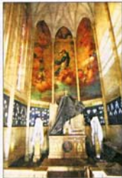
Holy site: A chapel awaits renovation.
